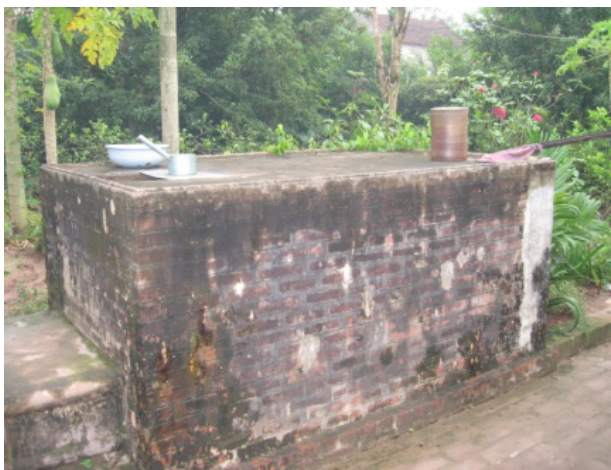
Rain water harvesting tank and pipe
