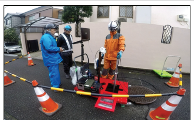
Figure 5: Operators working from above ground in UAV inspection.
